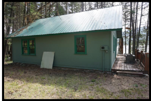
West Side of Building
