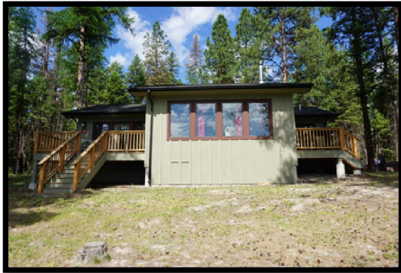
East Side of Residence
