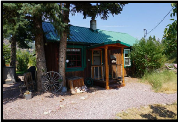
Cabin Entrance on South Side
