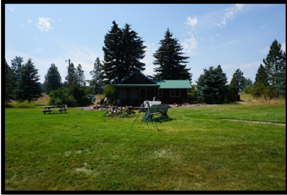
Front of Cabin on Lot 9 Looking West
