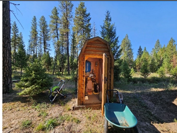
View of pumphouse behind the house.
