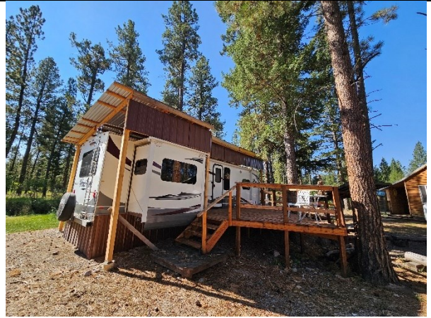
View of the covered RV carport and deck.
