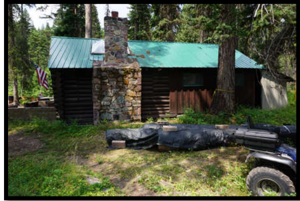
East Side of Residence
