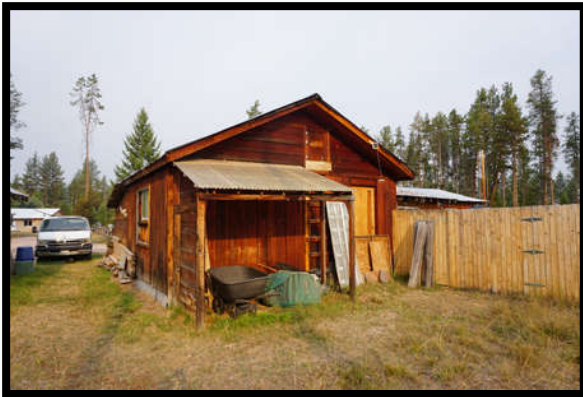
East Side of Storage Building
