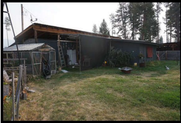
Residence and Fenced Yard on Lot 48
