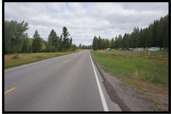
MT Highway 83 Looking North
