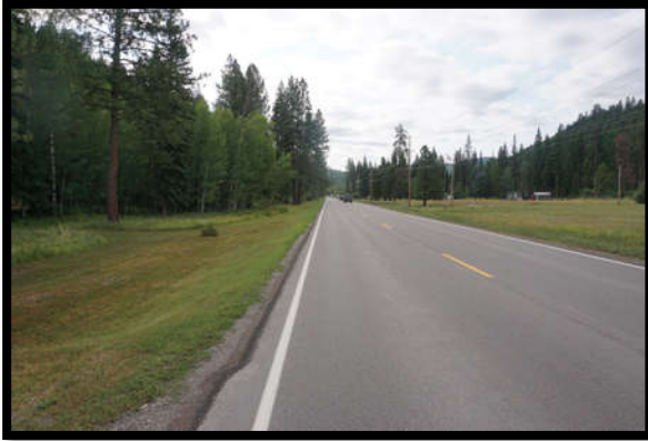
MT Highway 83 Looking South
