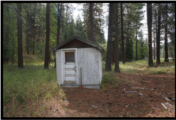
Well Pump / Storage Building on Property
