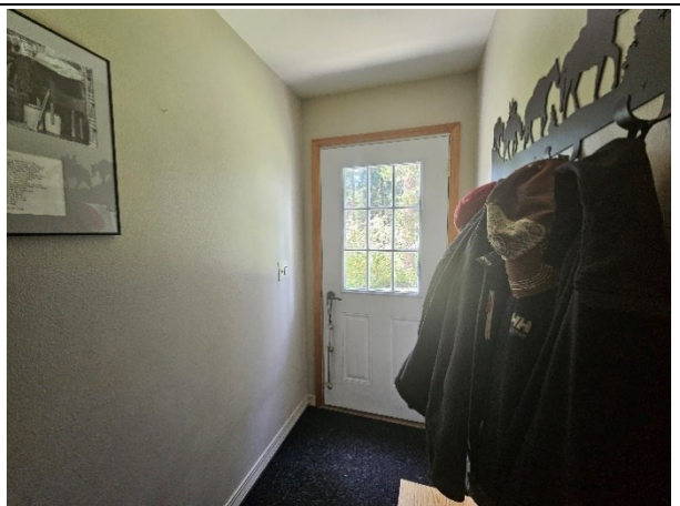
Interior view of the entrance on the west side of the SFR.
