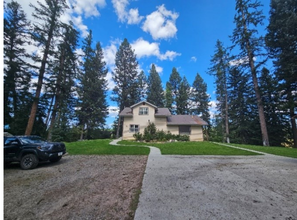
Rear elevation of the SFR.
