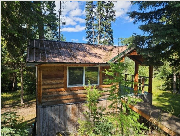
View of the bunkhouse from the access point from the front yard on the easterly side
