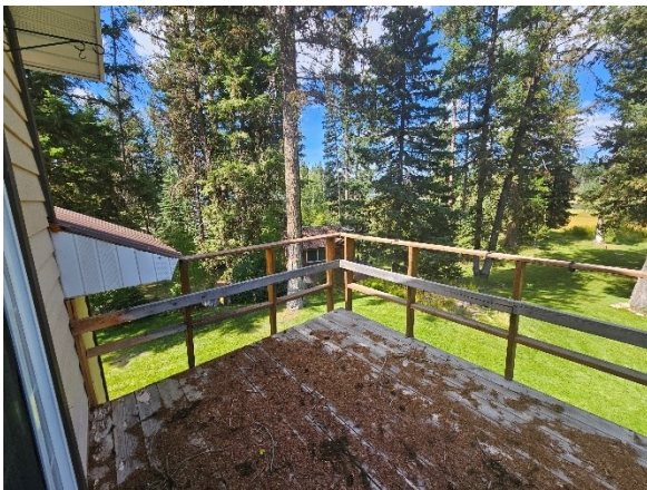
View of balcony off the primary bedroom.
