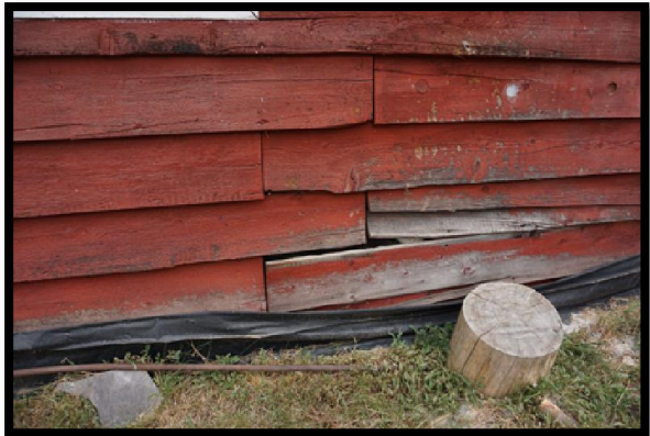
Siding Deferred Maintenance
