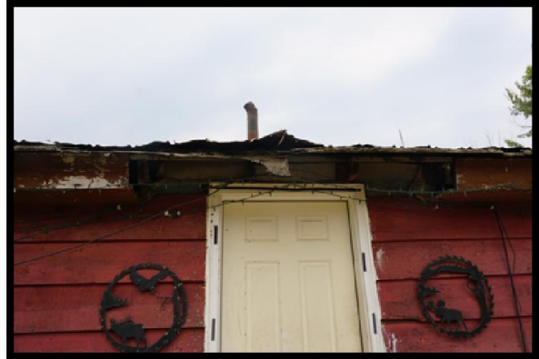
Fascia and Roof Deferred Maintenance
