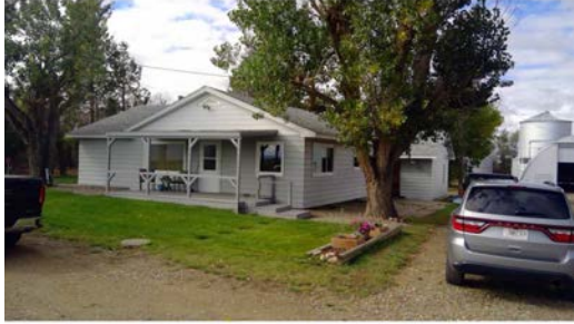
Dwelling Exterior Front
