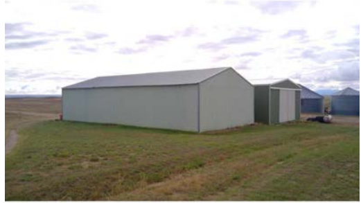
Implement Shed and Pre-Fab Building Rear
